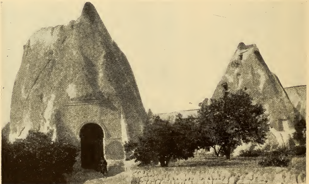
THE FACADE, DOORWAY, AND VESTIBULE OF THIS CHURCH ARE STILL WELL PRESERVED
