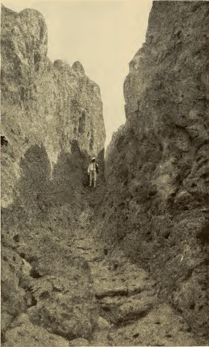
THE ENTRANCE TO THE VALLEY OF ORTAKIEUI (SEE PAGE 328) FROM THE PLATEAU IS ARTIFICIAL, CONSISTING OF A ROADWAY EXCAVATED THROUGH THE RIM-ROCK OF THE BLUFF
